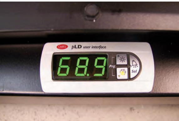
Temp Display and Setpoint Interface for SmartAire & PowerAire
